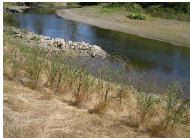
Streambank stabilization with stream bars and riparian re-vegetation in Oregon. (Photo by K. Boyer, USDA NRCS)
